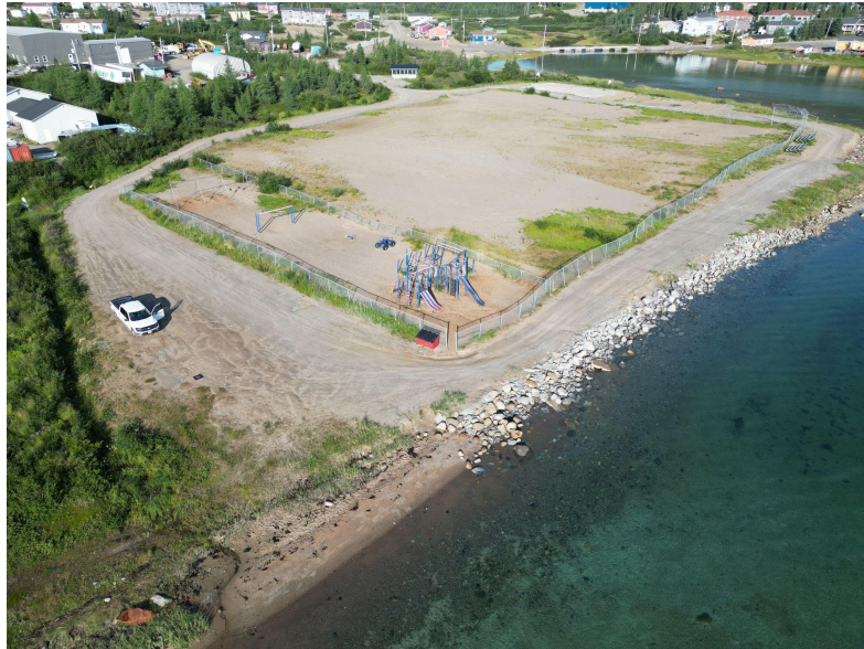
Figure 5.2: Oblique photo of region 4 collected with an uncrewed aerial vehicle. Differential subsidence is evident along the fence line of the park near the play structures.
